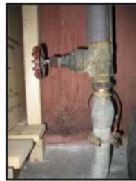
Examples of lead piping. Though lead is remarkably useful, it is also highly toxic.
