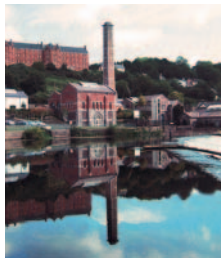
In 1997 Dan was appointed by Cork Corporation (now Cork City Council) to convert the Old Water Turbines into electricity generators for supply to their many electricity accounts.
