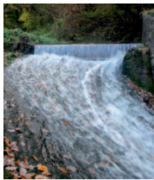
Dan utilised the fall and flow from the Lackloun River adjacent to his home to convey the water from the high point, through water pipes, to the turbine house.
