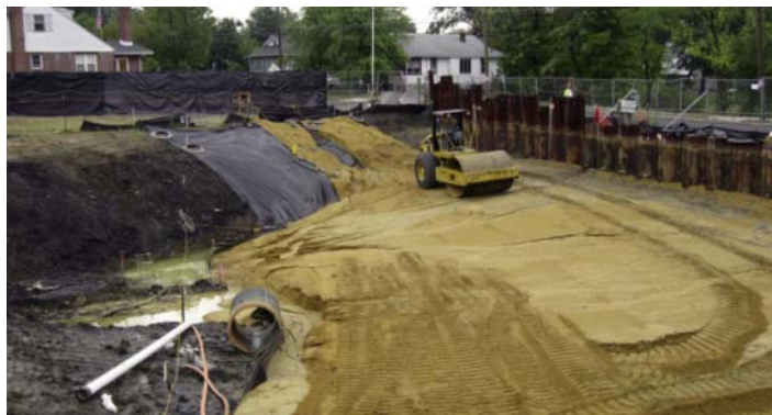
Backfilling the excavated soil with clean fill.
