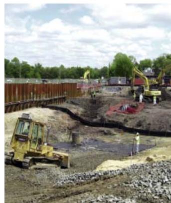
Removing contaminated soil.
