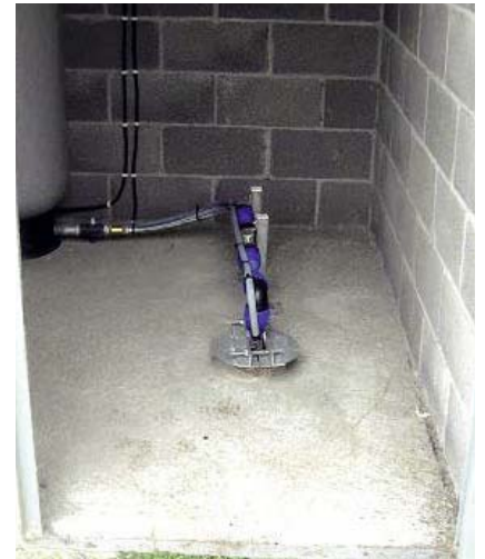
Figure 4: An example of a sealed and protected wellhead/borehole (Source: EPA)
