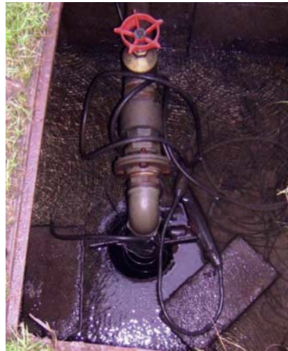
Figure 3: Poorly constructed wellhead with surface water entering the top of the borehole (Source: EPA)
