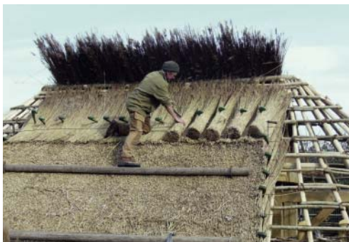
Applying the bundles of reed. The Thatch is imported Polish reed. This is the only element that had to be imported for the sad reason that most Irish reed beds are now so polluted with vibrates that the reed has grown too quickly and is weak and short-lived.
