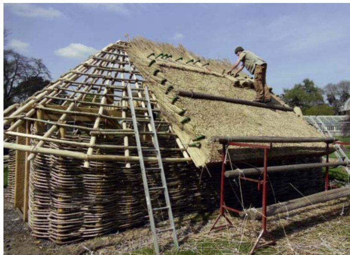
Peter begins the roof. The Thatcher uses a pole mounted between 2 boom hooks as his movable scaffold. The boom hooks are nicknamed 'Tritelas' in Denmark because of their resemblance to a 3. The hook penetrates the thatch and rests upon a rafter and is then hooked up behind the next higher rafter on the roof - an ingenious and easily moved support.
