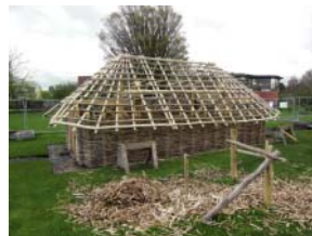
The roof batten out. The roof rafters and battens are made from Ash, either in the round or split lengthwise.
