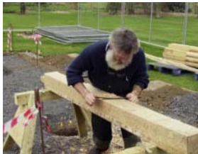
Eoin preparing the house posts.
