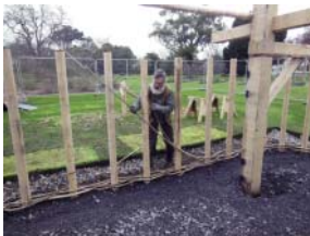
Beginning the wattle walls. The wattle walls are made from hazel rods.
