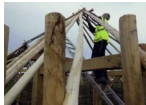
Beginning the roof.
