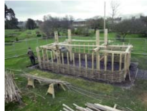
Walls half way up. The trestle supports are made from Oak, as are the house posts.
