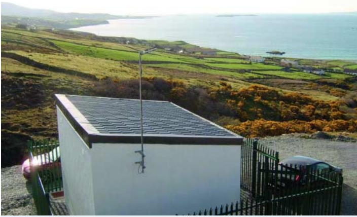
Lettergesh/Mullaghloss GWS (group water scheme) on the western fringe, near Killary harbour in north Connemara is typical of modern community-owned treatment plants that must meet national and international water quality standards. As with the vast majority of group water schemes, it is universally metered, householders paying for every drop of water they use beyond a 'free allocation' that varies depending on the financial circumstances of the scheme.
