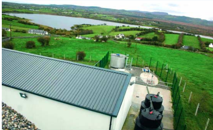
In the 1970s, the GWS sector expanded in lakeland districts of the West and the border counties, where scheme tended to be larger and supplied by gravity from reservoirs. Parke GWS (pictured above) is typical of many such schemes. The proliferation of isolated dwellings with septic tanks and intensive agriculture around the lake source has contributed to nitrification of the source and consequent algal blooms that increase the cost of treatment.
