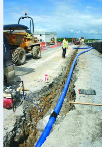
Because of the dispersed population in rural Ireland, distribution networks are proportionately much longer per household than on public supplies. Pictured above is the laying of a new network on the Mid Roscommon supply.
