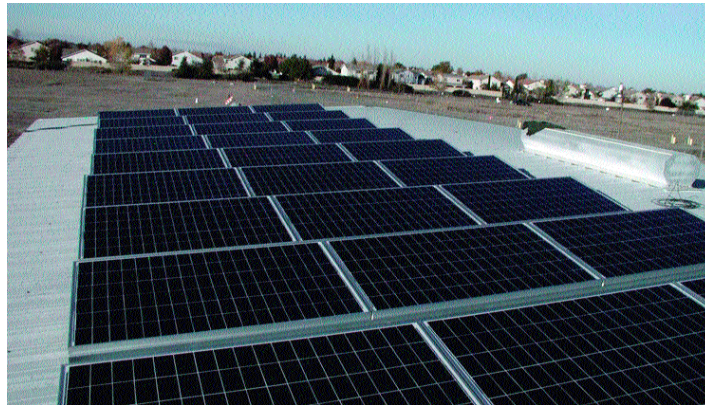
This site was the location of Brockton Gas Works, Brockton, Massachusetts, from 1989 to 1963. The potential for contamination meant it was designated a brownfield site, so it held little appeal for redevelopment. Following remedial activities and capping, the site was turned into a useful, renewable energy source with the installation of approximately 1,400 solar panels, providing 425 kilowatts of electricity directly into the local grid each day.
