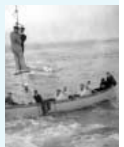
A bosun's chair, used to hoist men on to or off stations where landing conditions were poor, as shown here at Fastnet.
