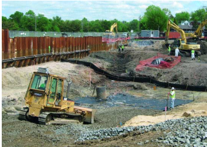
The Welsbach/General Gas Mantle Contamination Site, located along the Delaware River waterfront, New Jersey, USA. Two former incandescent gas mantle manufacturing facilities used the radioactive element thorium in their manufacturing process, which has contaminated the site. Part of the clean up involves excavation and off-site disposal of radiologically contaminated soil and waste materials.
