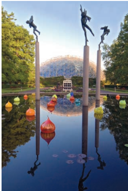
THE CLIMATRON – One of the most recognizable icons of the Garden is the Climatron conservatory. It was the first geodesic dome to be used as a greenhouse. Built in 1960, the structure, designed according to the principles of R. Buckminster Fuller, rises 70 feet in the centre with no interior support, allowing more light and space for the half-acre of tropical plants within.
