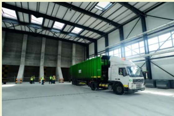
A truck in the tipping hall.
