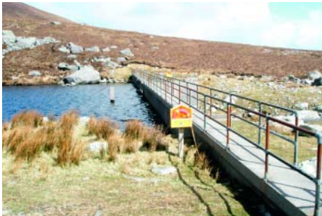
Significant alterations to the lake outlet, such as this dam at Accorymore Lough in Mayo, results in an otherwise high status lake being downgraded to good status.
