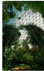
THE CLIMATRON – One of the most recognizable icons of the Garden is the Climatron conservatory. It was the first geodesic dome to be used as a greenhouse. Built in 1960, the structure, designed according to the principles of R. Buckminster Fuller, rises 70 feet in the centre with no interior support, allowing more light and space for the half-acre of tropical plants within.
