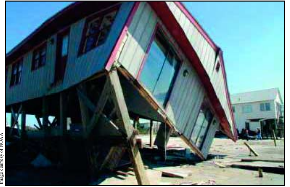
Homes built too close to shore can be destroyed by waves during storms.
