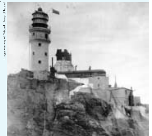
The new Fastnet tower, off the coast of Co. Cork, and the remains of the old tower being dismantled.
