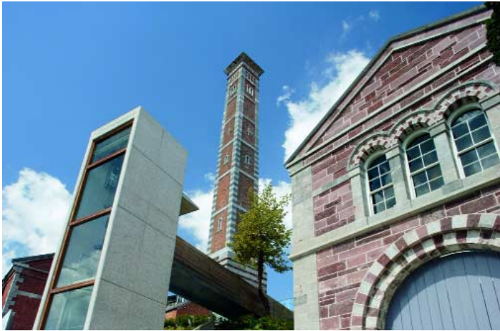
Lifetime Lab entrance at Old Cork Waterworks.
