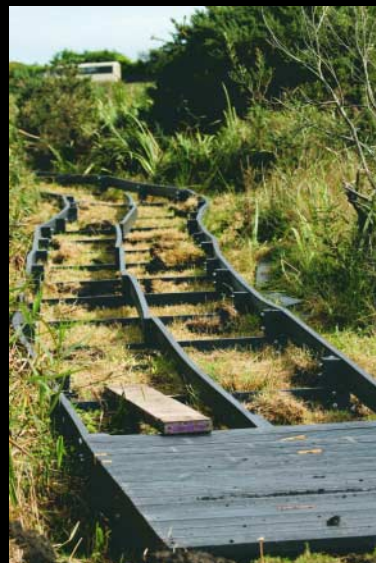
Constructing a boardwalk.
