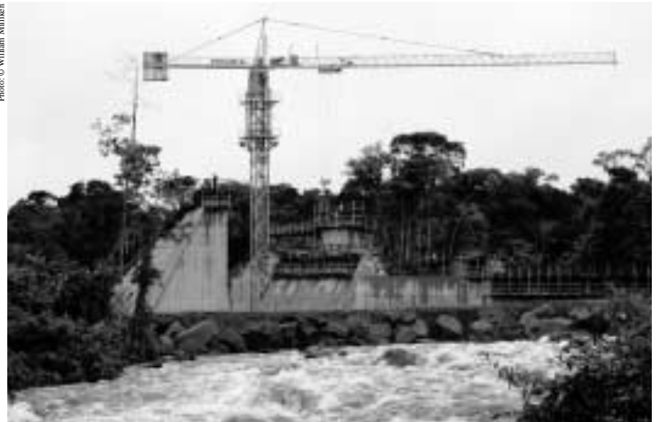
Constructing the new Rochedo hydroelectric dam in Mato Grosso State in the Brazilian Amazon. Can the biodiversity impacts of such projects really be offset?
