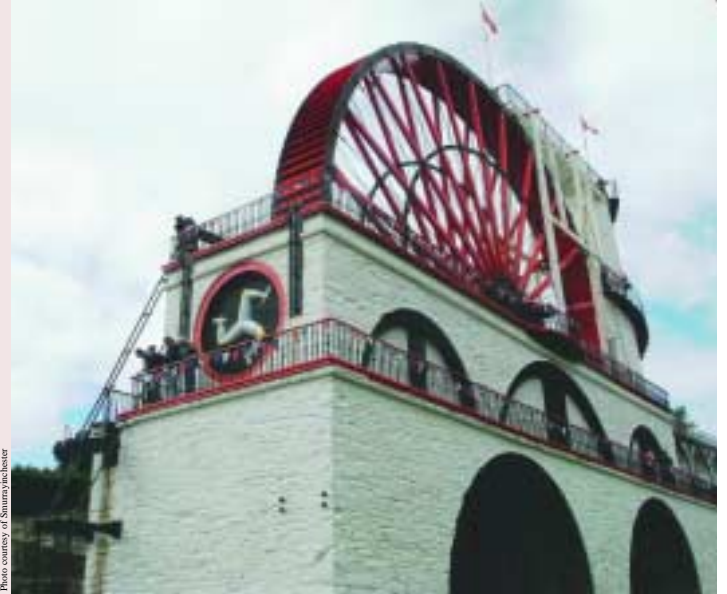
The Lady Isabella, Isle of Man: a huge water wheel, once used to remove water from a mine.
