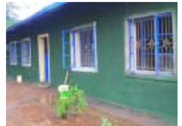
A classroom on completion.
