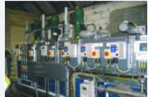
The pilot treatment plant which was in place in Avoca for three months in 2006.
