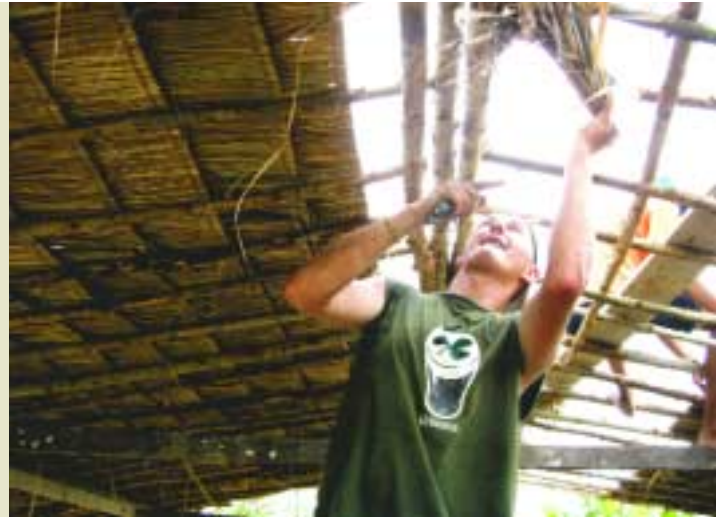
One of the group working on the roof.
