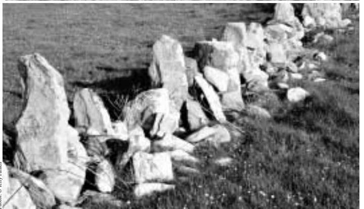
Top - A carefully built wall is both functional and surprisingly stable. Above - Though walls may collapse over time, they can be easily rebuilt using the fallen material.
