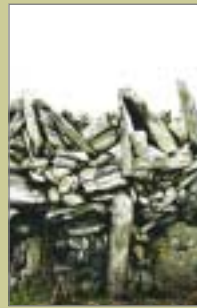
Above left: The underlying geology can influence the building style of a wall. Above right: Infilling with small stones at the base presents a barrier to small animals.
