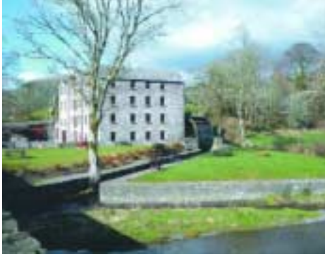
Restored Corn Mill, Macroom, Co. Cork.
