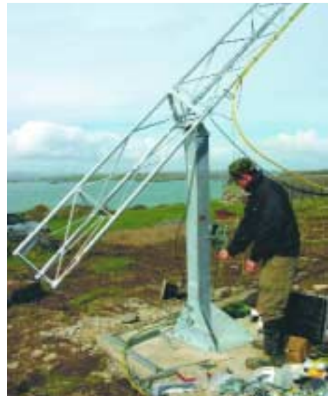
Howard fixing cables to the mast from the anemometer sensors on top.
