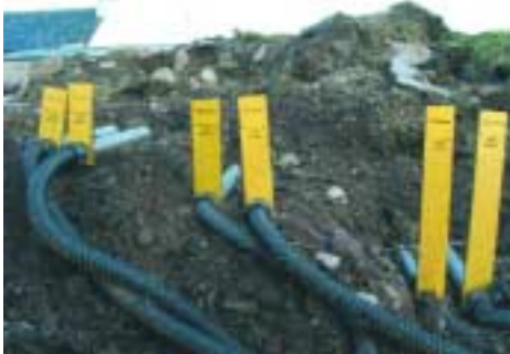
The Soil PRT (thermometer) pairs with their depth gauges fitted, before being covered in.
