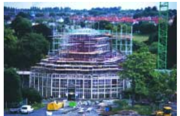
Scaffolding in place to begin restoration
