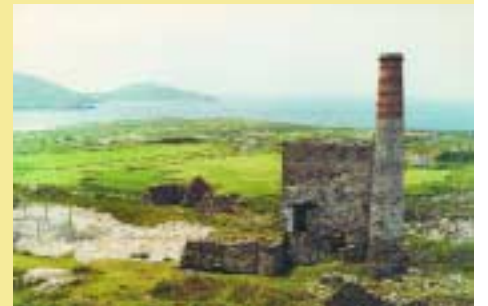
Allihies, Co. Cork. Engine house and Cornish chimney looking out towards Dursley Island.
