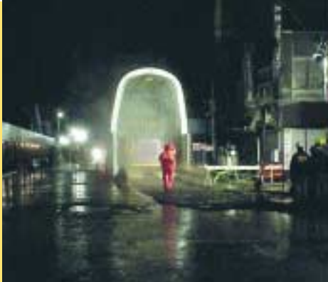
A wash station to wet down and decontaminate trucks taking debris to barge sites
