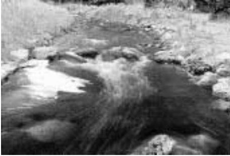
Picture: a vortex rock weir concentrates the flow to the centre of the pool, creating depth and providing cover.
