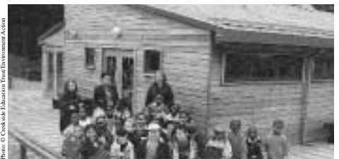
High flier's overhead: Deptford's wooden-framed education centre is fitted with a "green roof", good for wildlife such as Black Redstarts.
