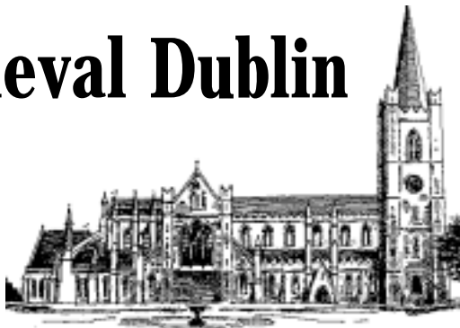
St. Patrick's Cathedral from the north. The Minot Tower dates from c. 1370 and its spire only from 1749. Much of the external fabric is modern.
