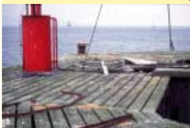
The timber section of the ESB dolphin, Dublin Port.
