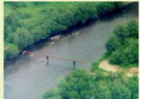
Gas pipeline crossing the Kol River. Will development follow?
