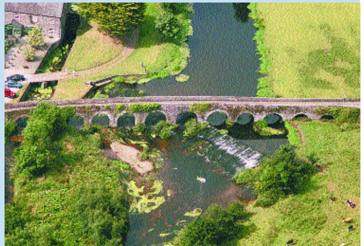
The ancient bridge over the river Funshion at Glanworth, Co. Cork, perhaps Cork's oldest surviving one.
