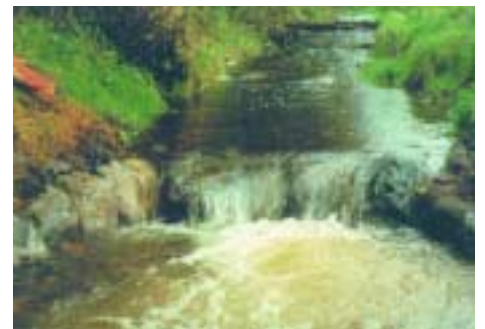
A stone weir has been provided in what was formerly a featureless stream. The weir provides depth, cover and natural oxygenation thus greatly improving habitat for juvenile trout and salmon.
