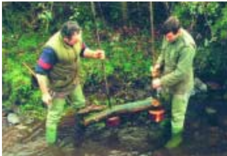
A natural log with "spacers" underneath is put in place in stream bed to provide cover and shade for young fish.
