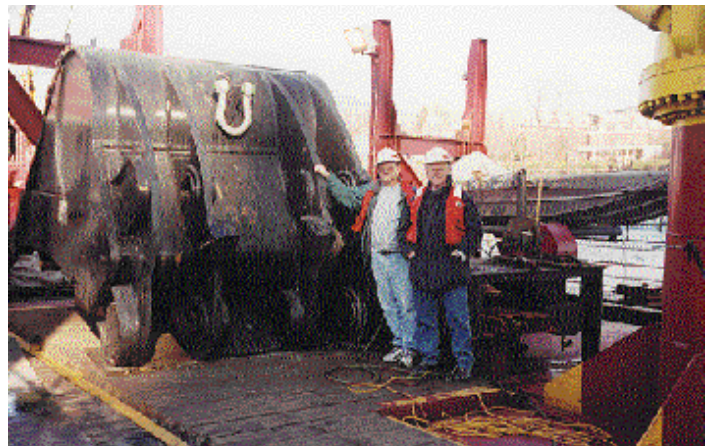
Michael Ludwig (left), the author and Matt Murphy (right), standing next to one of the power shovels that removes unpolluted sediment to deepen the harbor. It has State-of-the-art electronics that allow precise removal at ten yards per bucket full.
