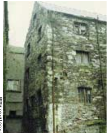
Fine masonry incorporating cut limestone, red sandstone and brick in a now demolished old building in Cork City.
