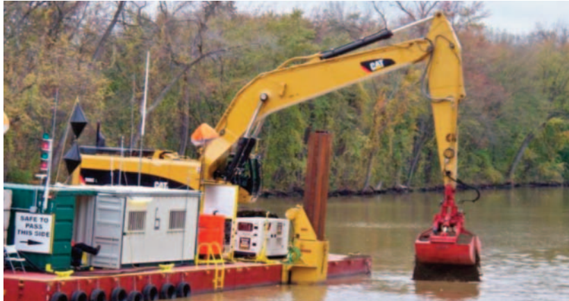
Dredging at the Hudson River PCBs Superfund Site
