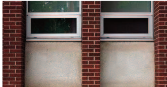
PCBs were used as plasticizers and stabilizers and extenders in paints, cement, caulk, floor finishes, pesticides, adhesives, waterproofing materials and much more.
