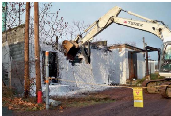
Radium vault demolition in 2008.
