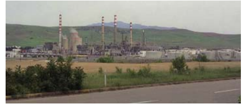
Technical Assistance on the Implementation Capacity of the Seveso II Directive in Turkey by AWN Consulting
