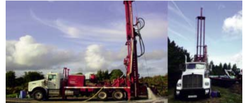
Two large Open Loop Geothermal wells in County Durham, UK by Meehan Drilling
