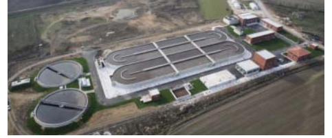
Construction, Supervision & Technical Assistance at Luluburgaz, Turkey. Elimination of pollution of the Eugene River and compliance with the EU Urban Wastewater Directive by J.B. Barry & Partners.
