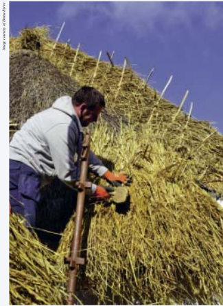
The thatcher working on the gable of Old Mill Cottage.
