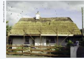
The straw goes on in layers and is held in place with twisted hazel stays or scollops. Once the front and back are completed, the thatcher's start on the sides, building up the straw as per the front.
