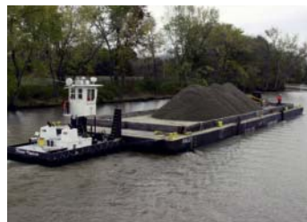
After an area has been dredged of contaminated sediment to the EPA's standards, clean backfill is transported on a barge by a tug boat. The backfill replaces dredged sediment and maintains the natural contours of the riverbed.
