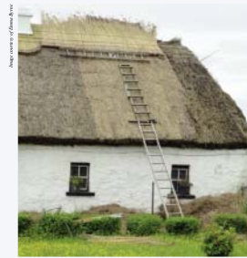
A thatching in progress. You can see the uncut reeds on the ridge and the difference in colour between the old and new straw.
