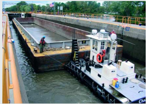
Tugboats are used to move barges of contaminated sediment to an upstream processing facility and clean backfill to the previously dredged areas. The tugboat and barge must navigate through the lock system to get to the processing facility. The barges may make as many as 20 one-way trips to and from the processing facility during a 24-hour period.
