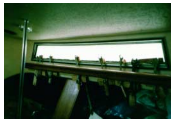
The window repairs after the knockdown.
