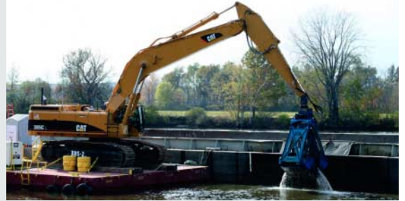
Workers use excavators with environmental clamshell buckets mounted on flat, anchored platforms to dredge the river. The PCB-contaminated sediment is emptied onto 35-foot-wide, 195-foot-long floating barges.
