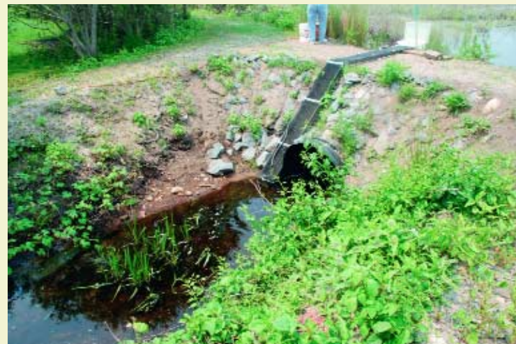
HCT volunteers count American eels that migrate over a dike, thanks to HCT's innovative eel migration ramp.
