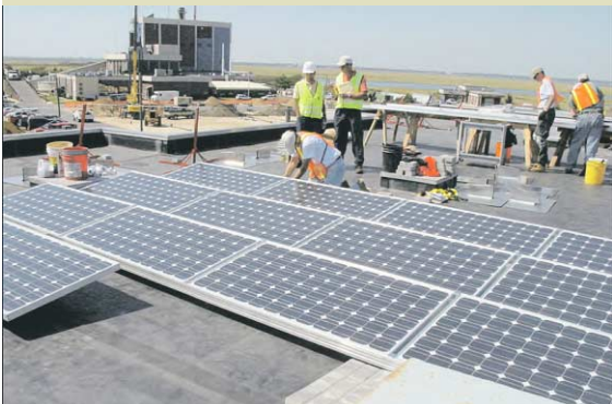
500 kw solar array at Atlantic City Municipal Utilities Authority sewage treatment plant (Atlantic City, New Jersey)
