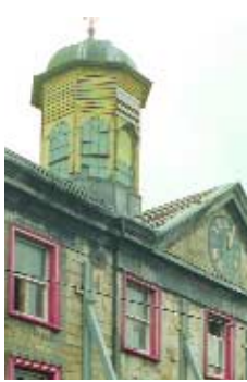
Hoarding covering the clock tower.
