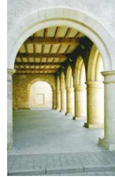
The restored arches.
