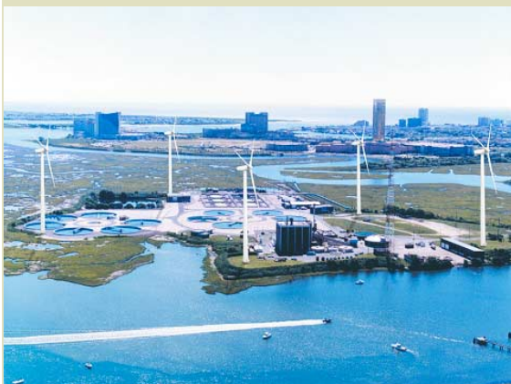
Five large wind turbines installed on grounds of Atlantic City Municipal Utilities Authority sewage treatment plant (Atlantic City, New Jersey)
