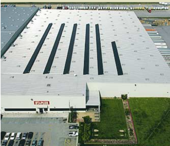
MW solar installation on roof of a "Staples" office supply store.
