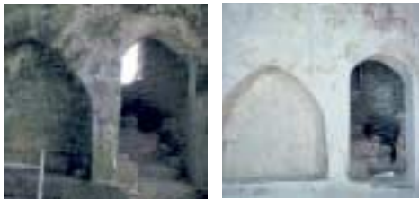
Above left: Algal growth on the Cistercian Abbey on the island. Above right: The walls were laboriously cleaned.
