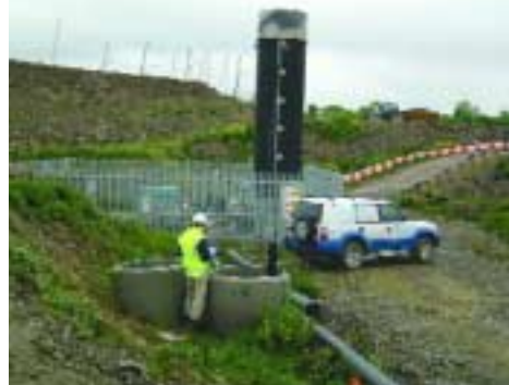
Landfill gas monitoring
