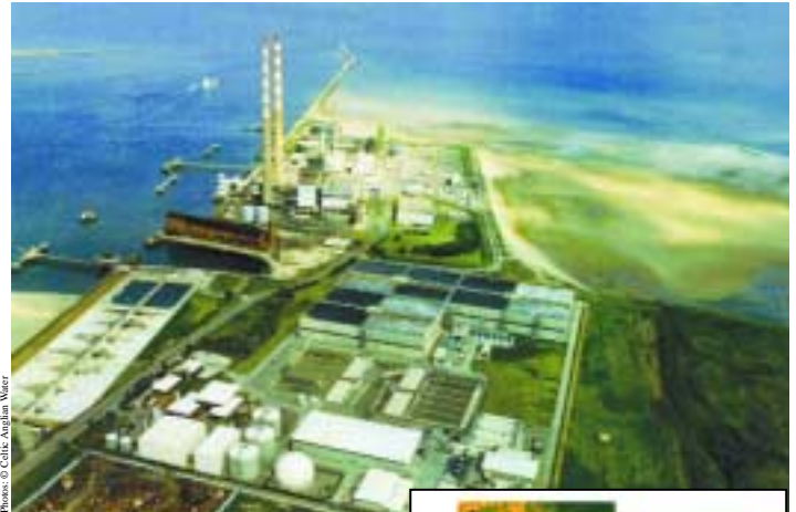
Ringsend Wastewater treatment works
