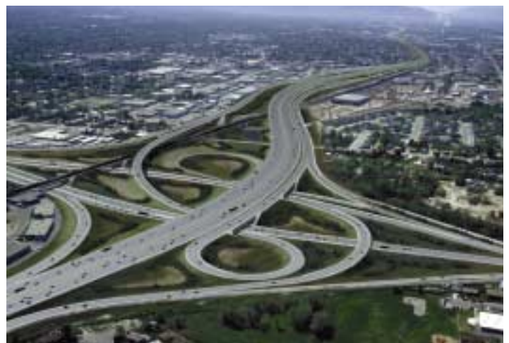
This major interchange in the US is a recent example of engineering excellence and cultural impact. Choices are defined and made through planning at a federal, regional, and local level.
